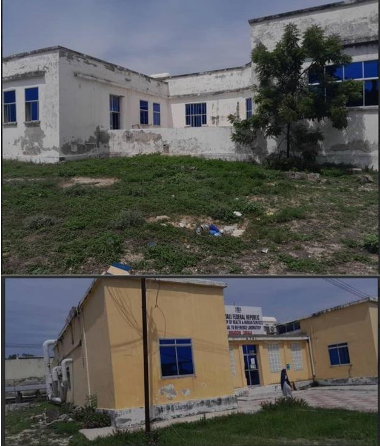
Figure 8 Photos of current state of Forlanini Hospital
