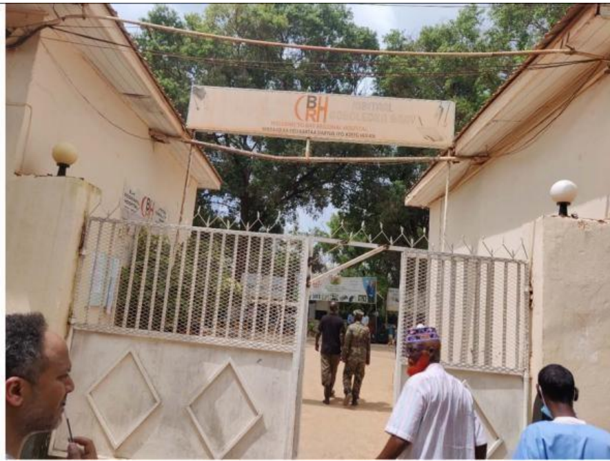
Figure 9 View of the existing building
