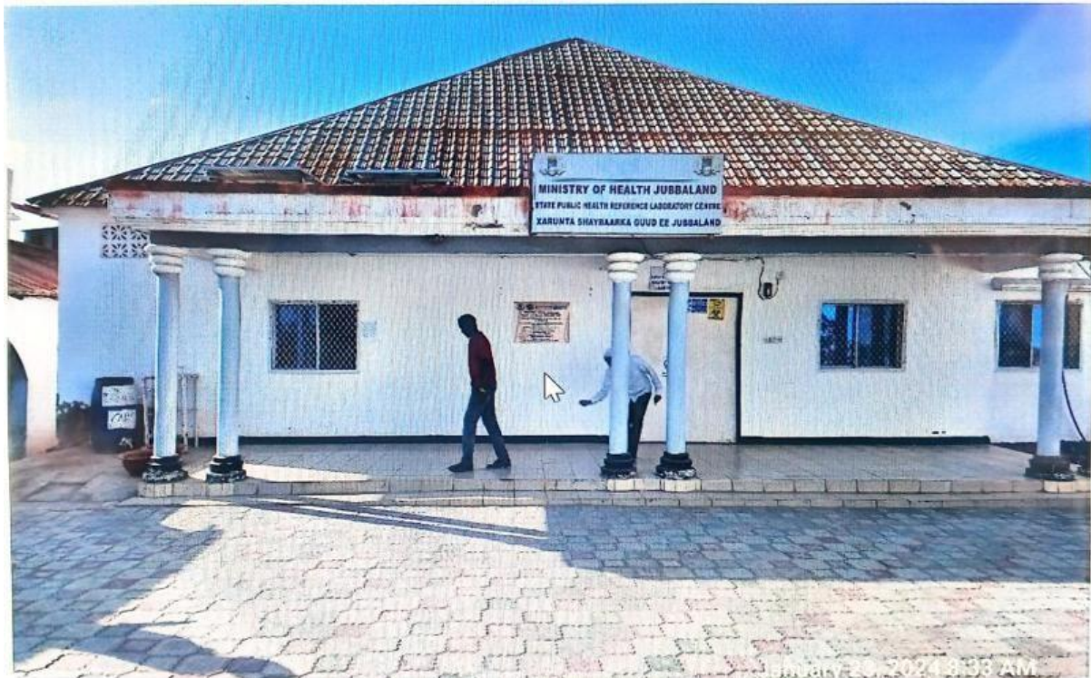
Figure 10 Existing Facility at Kismayo Hospital
