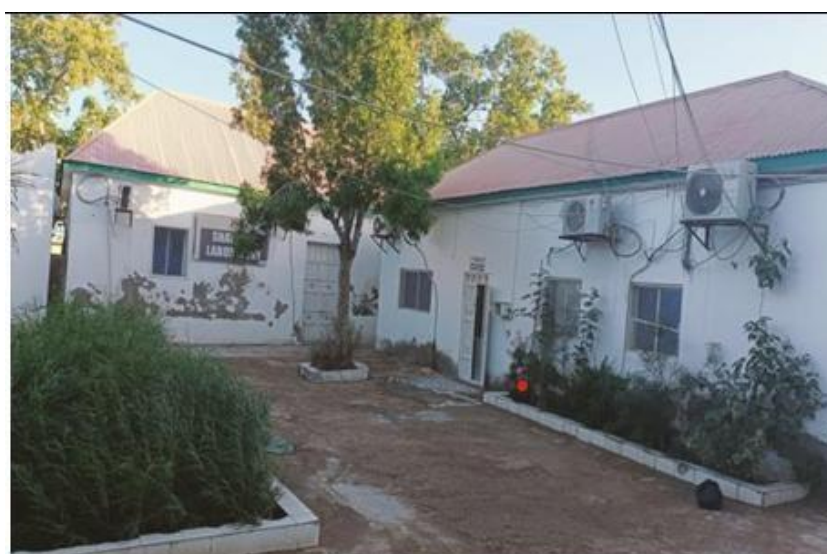
Figure 9 Existing Facilities of Bosaso Hospital
